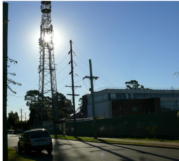
Figure 10 Carlingford Electricity Substation The electricity substation is located north of the subject site at the corner of Jenkins and Felton Road.
